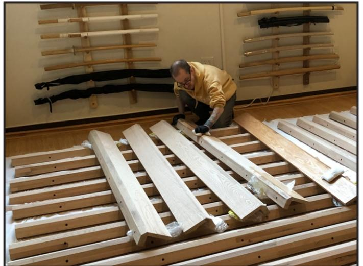
The second delivery of materials was made on Friday, February 24, and consisted of the subfloor components. Assembled, the subfloor is two layers of 1/2-inch birch plywood. The bottom layer comes with six-inch, steel springs attached— pieces to be placed on the outside edges of the subfloor have double the number of springs along the edge(s). In total, our system has almost 1,500 springs.
